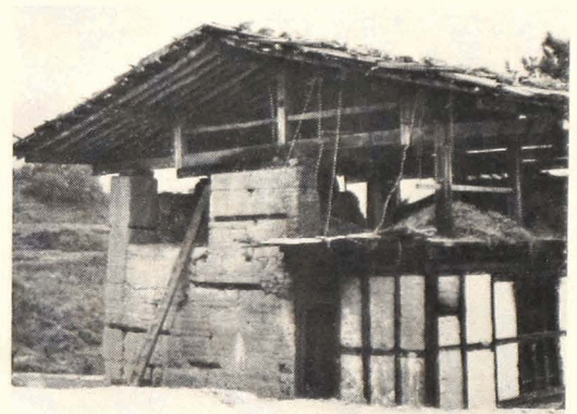
3. Roof details of a farmhouse.
